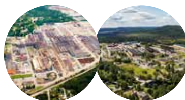
Hofors & Hällefors Ingot based casting of highest quality clean steel
